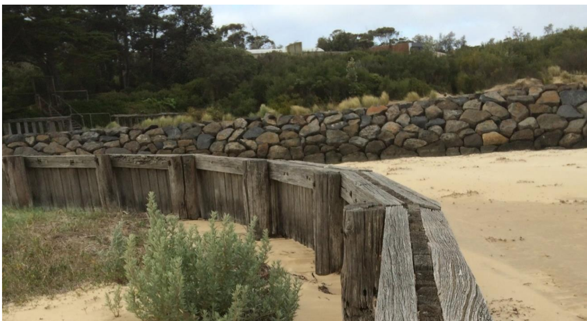
Figure 9. Rock wall and timber structure, looking across mouth from west to east (old timber structure on west side of estuary in foreground, with new rock wall on east side in the middle ground) (Source: Alluvium, 2015)
