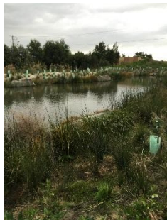
Asset 80 Plants failing to establish in newly constructed wetland given no apparent flow management during establishment phase
