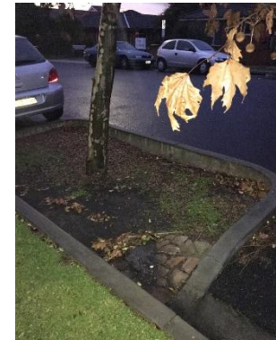
Asset 65 Surface level of filter media higher than inlet level
