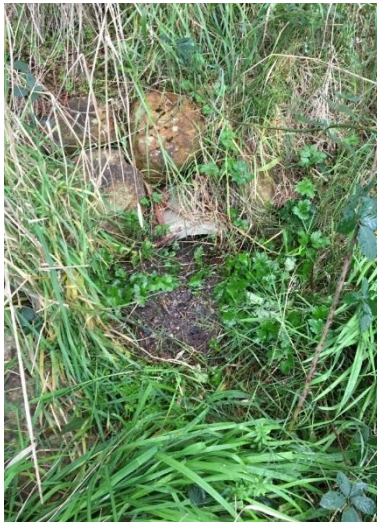
Asset 86 Completely blocked inlet
