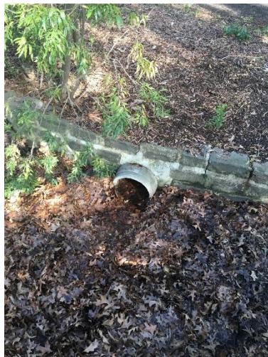
Asset 83 Partially blocked inlet
