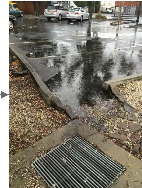
Asset 33 Overflow pit level flush with inlet level
