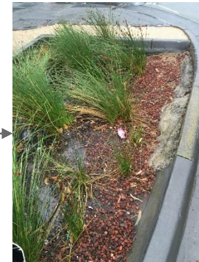
Asset 50 Surface not flat – some area not engaged
