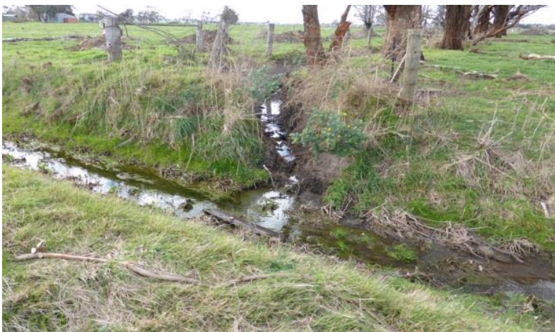
Figure 6: Private drain intersecting a Precept Drain
