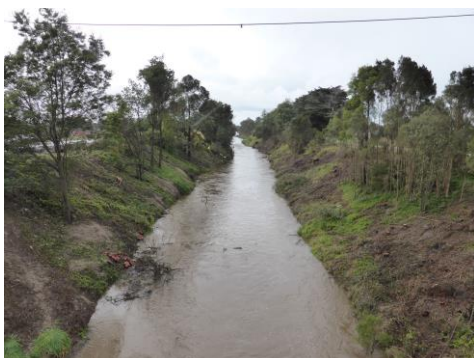
Figure 4: Bunyip Main Carrier Drain
