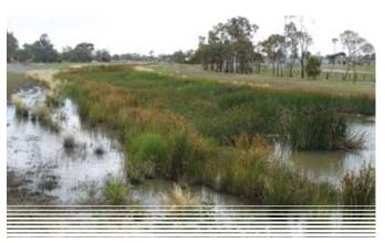
**Figure 5** After – following waterway rehabilitation works. The constructed waterway has a more natural form, with improved habitat and water quality treatment.
