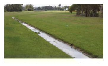
**Figure 4** Before – a grassed floodway with a concrete-lined channel that has very limited ecological value.
