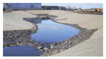
Figure 17 Waterway re-alignment, showing jute-matted banks prior to planting.
