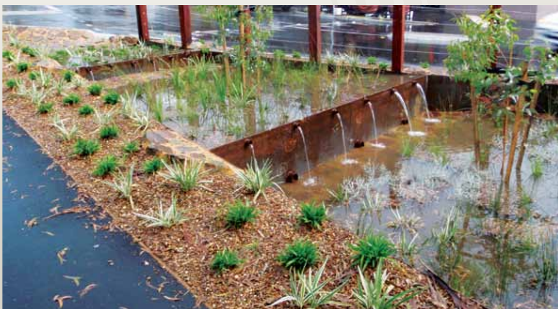
Were Street Raingarden constructed by Banyule City Council with support from Living Rivers Stormwater Program
