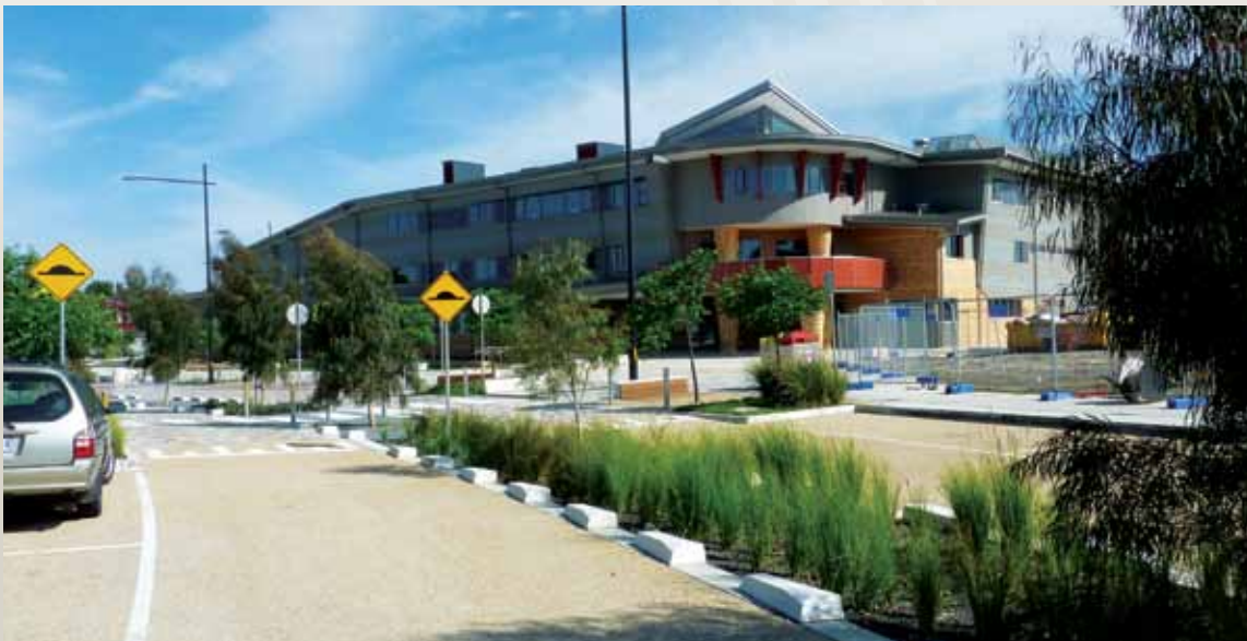
Tanderrum Way, Broadmeadows is one of many projects delivered in partnership with local government.
