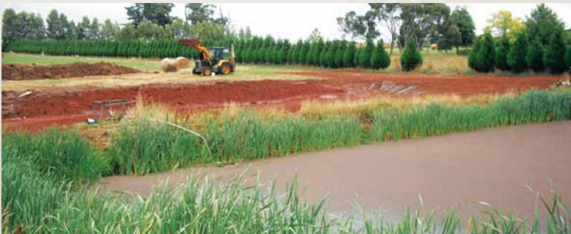
The wetland during construction
