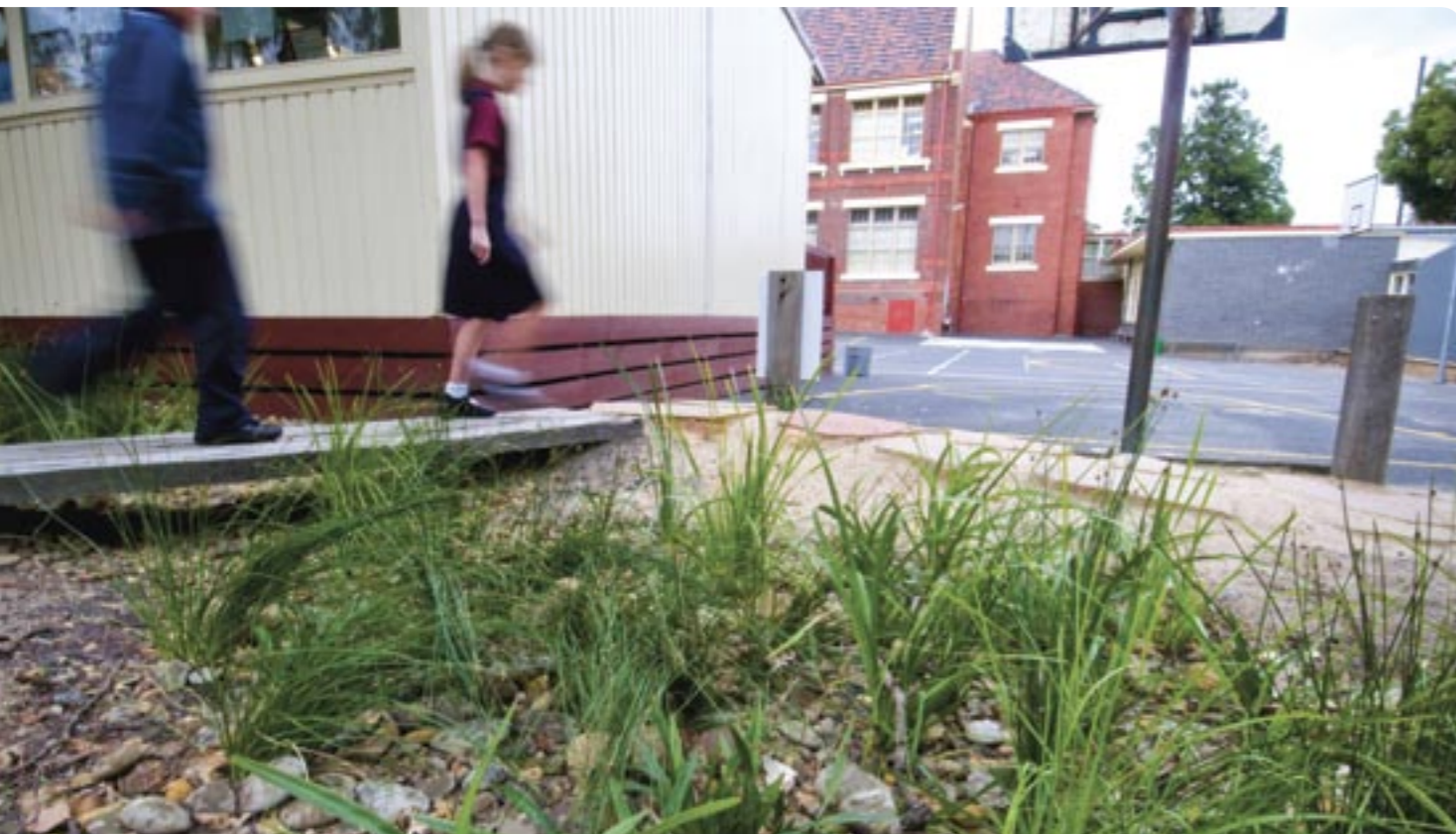
Raingarden at Toorak Primary School
