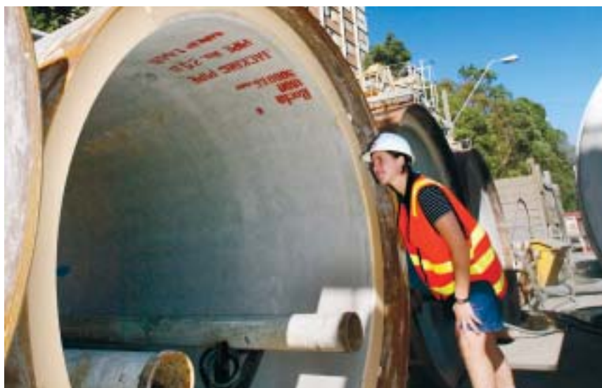
Contractor Zoe Bozinis inspects progress on the upgrade of the Palmer Street diversion drain in Richmond.
