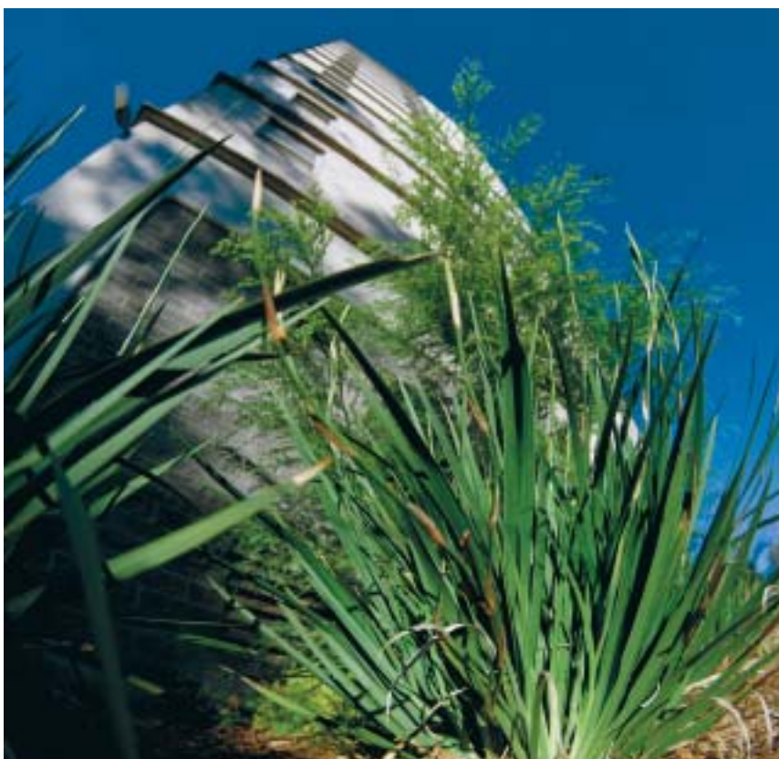
Melbourne Water and the Office of Housing are working in partnership to deliver an innovative stormwater recycling project at the King Street housing estate in Prahran.
