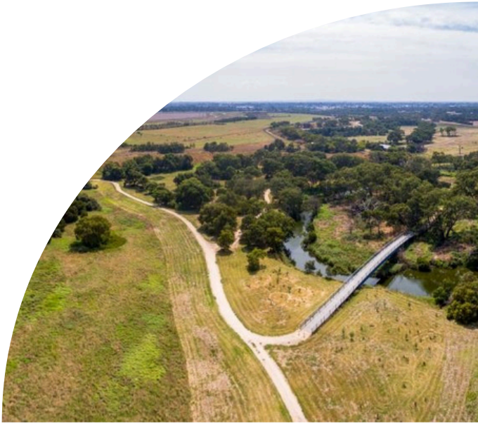
Aerial view of the Pedestrian Bridge at Werribee River Regional Park and surrounding vegetation before flood damage. Photo courtesy of Visit Werribee
