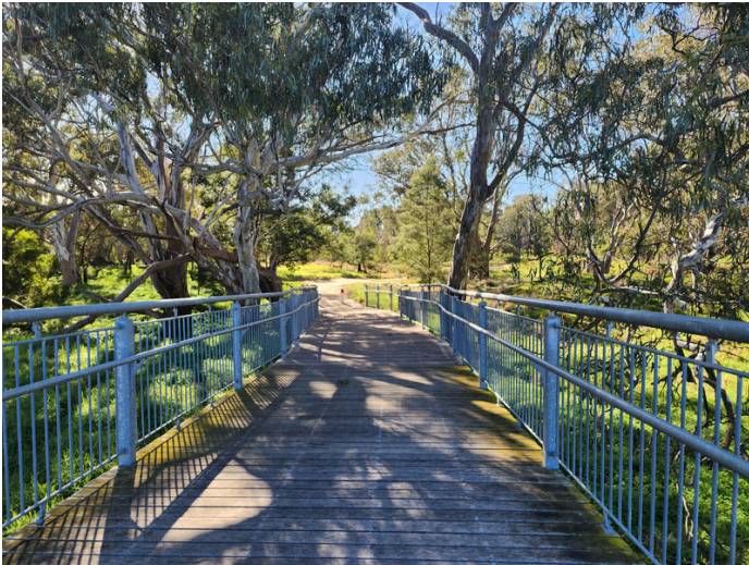
Werribee River Regional Park pedestrian bridge. Photo courtesy of Susanne Jensen, Werribee River Association.
