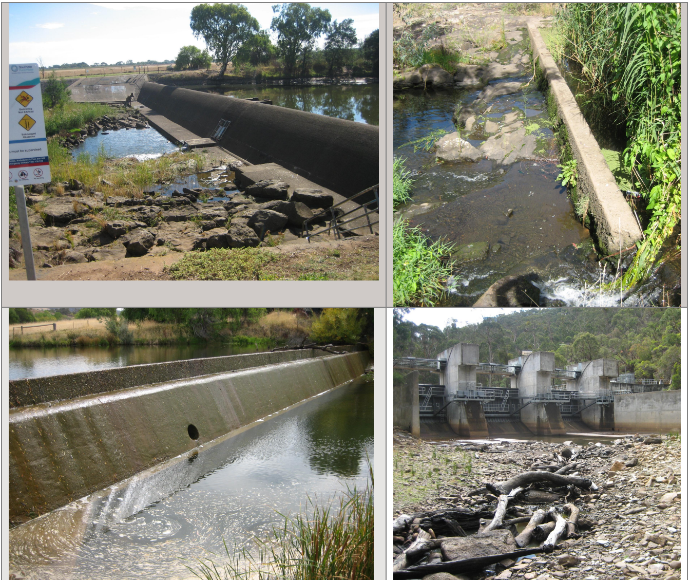
Figure 9-1: Examples of fish barriers in the Werribee River catchment. Top left – Lower Diversion Weir (Werribee); Top right – small concrete barrier downstream of Bungeys Hole; Bottom left – Upper Diversion Weir (Bacchus Marsh); Bottom right – Lerderberg Weir (this structure has a vertical slot fishway to assist fish passage).
