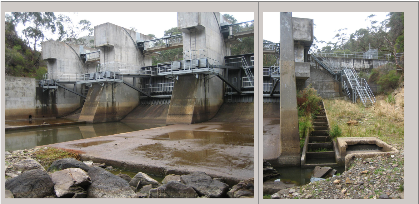
Figure 9-2: Lerderderg Weir (left) and vertical slot fishway (right)
