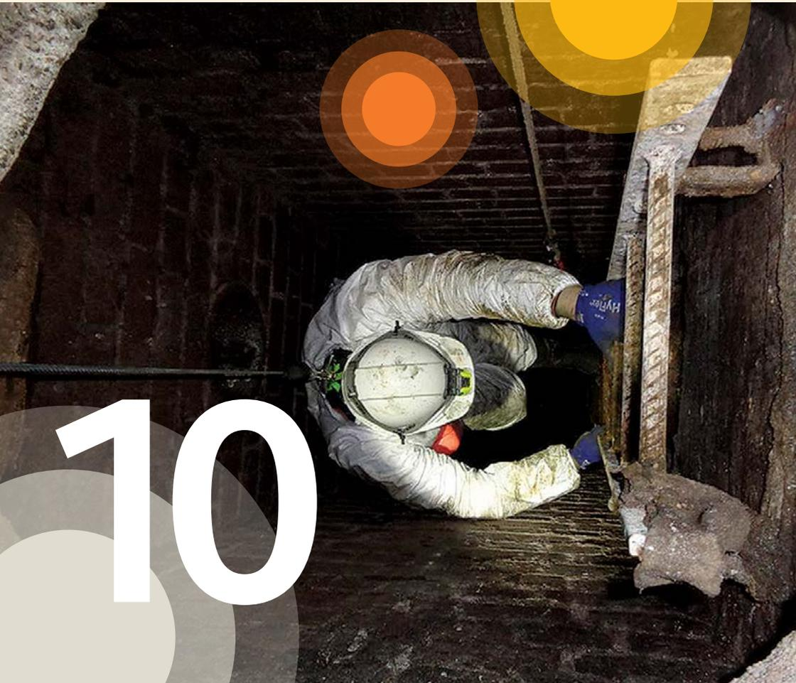
**The Sewer Transfer Operations Team are responsible for managing safe entry and exit to the 400 kilometres of Melbourne Water’s gravity sewers.**
