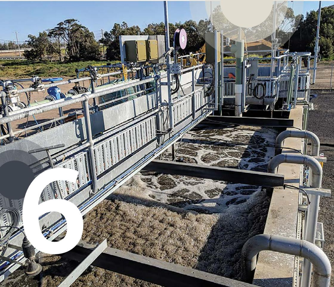
**Nitrogen removal, a vital step in the sewage treatment process at the Western Treatment Plant (WTP), reduces nutrients in the treated water discharged to Port Phillip Bay.**
