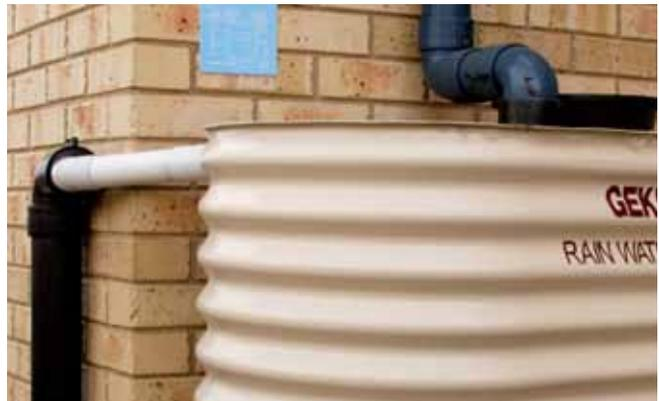
Rainwater tanks collect roof runoff for subsequent reuse, conserving potable mains supplies and reducing stormwater runoff volumes and pollutants from reaching downstream waterways.
