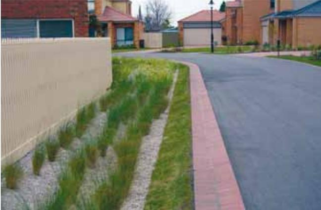
Bioretention swales (or bioretention trenches) are bioretention systems that are located within the base of a swale. They provide both a conveyance function for stormwater and treatment through filtration, extended detention and some biological uptake. The swale facilitates the removal of coarse to medium sized sediments, while the bioretention system is particularly efficient at removing nitrogen and other soluble or fine particulate contaminants.
