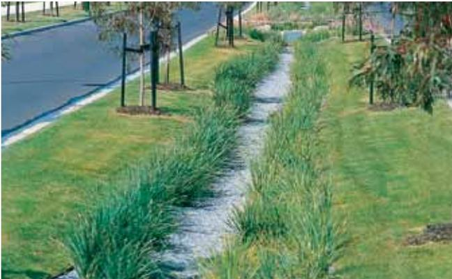
Vegetated swales convey stormwater and provide removal of coarse and medium sediment.
