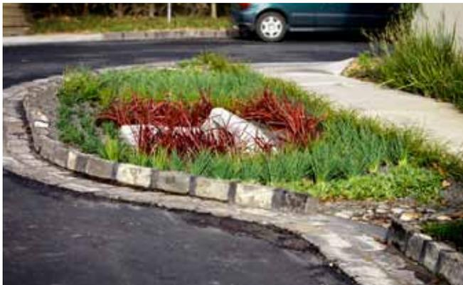
Bioretention basins and rain gardens treat stormwater by passing runoff through prescribed filter media (commonly vegetated) that provides treatment through fine filtration, extended detention and some biological uptake.
