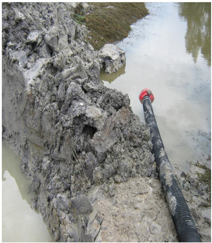
Figure 4: Sediment pond being manually pumped down
