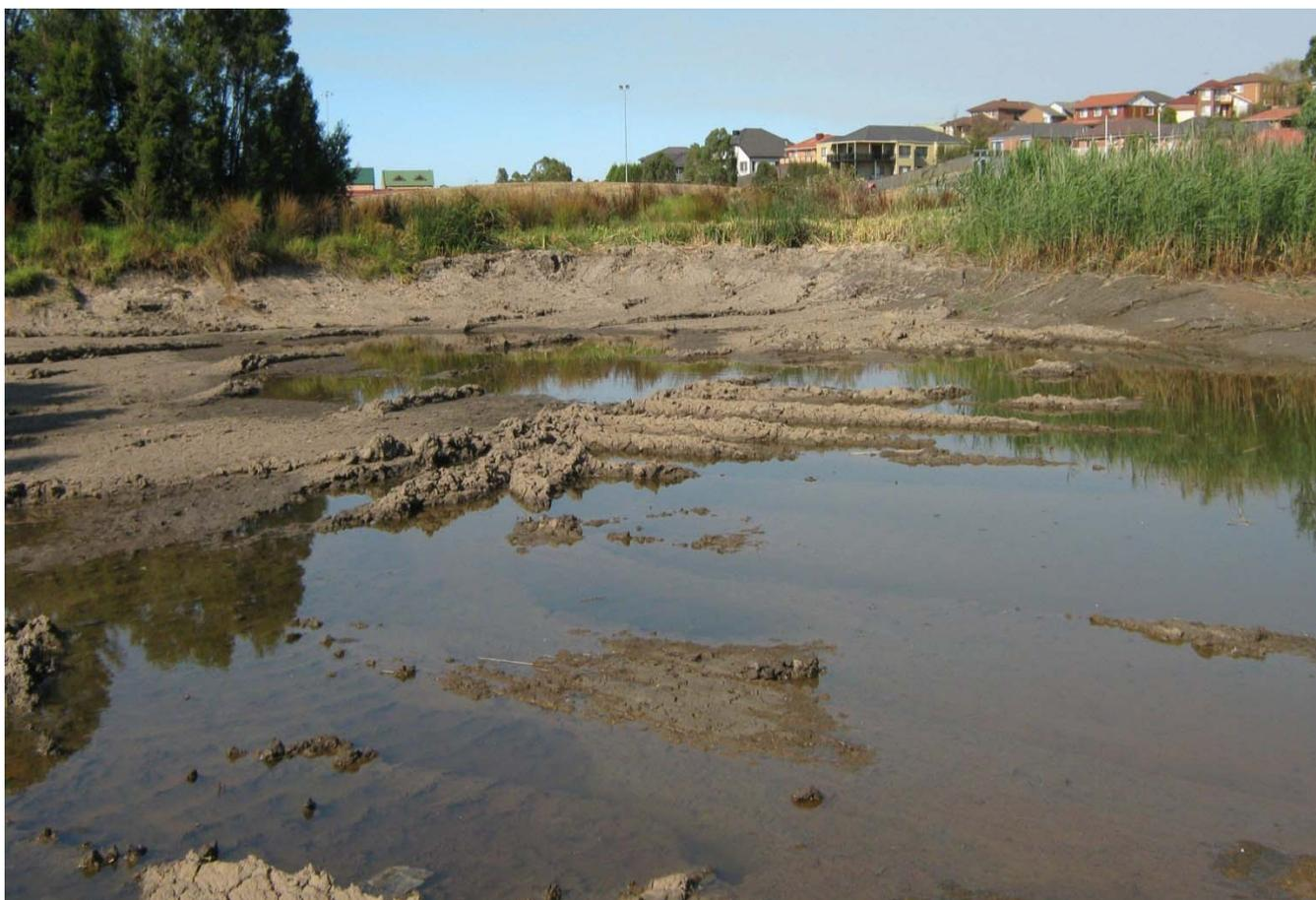
Figure 14: Sediment pond base prior to rock lining
