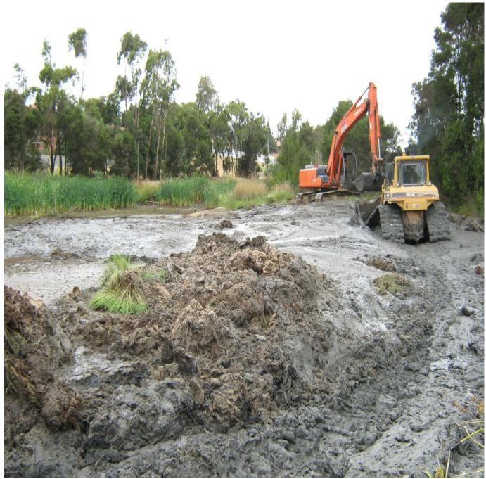
Figure 8: The swamp dozer pushes the semi dried material over to the excavator.
