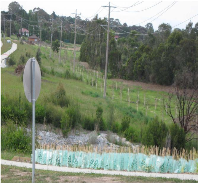
Figure 16: Reinstated sediment pond edge planting & rock work
