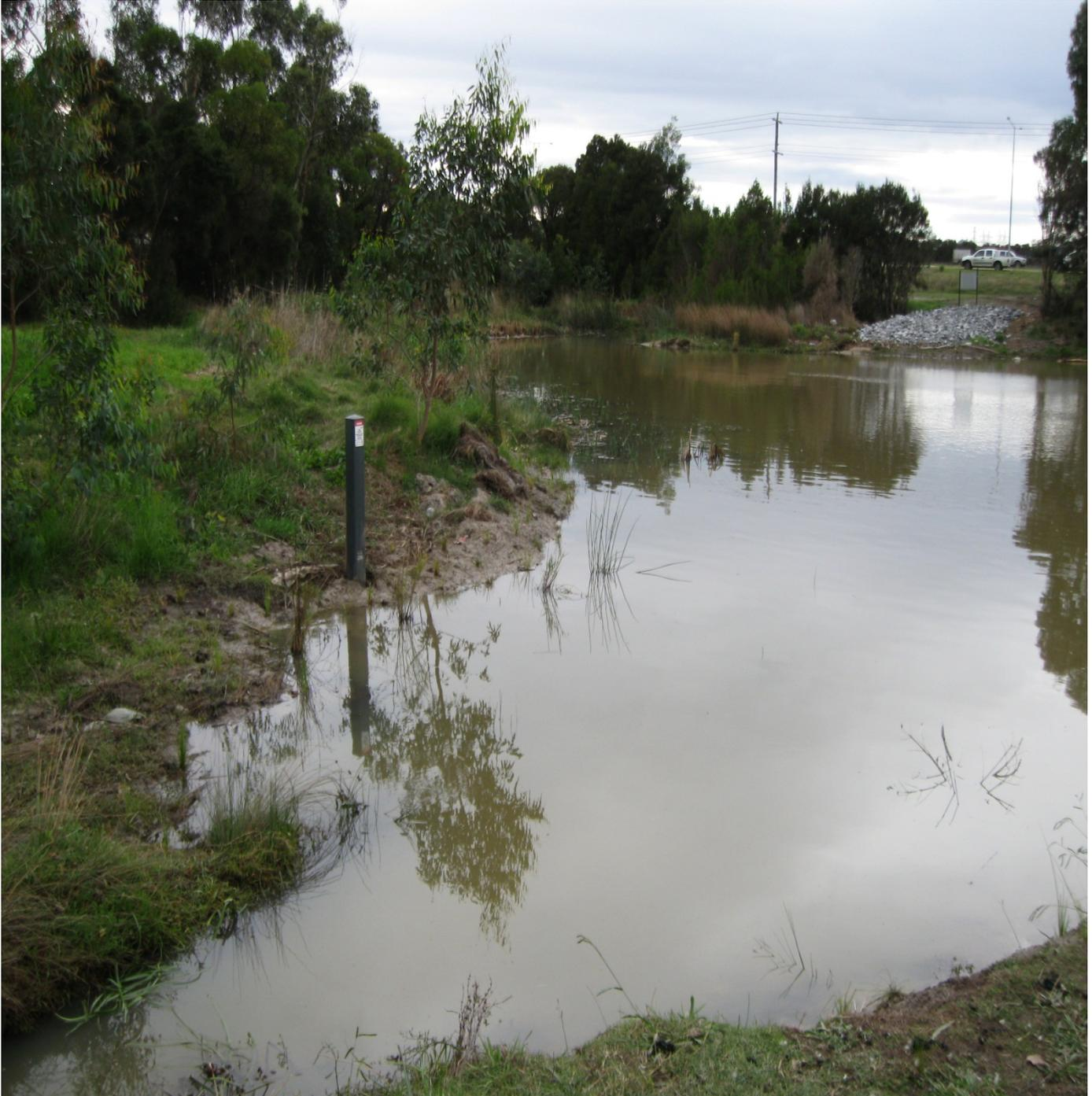
**Figure 3: Sediment pond prior to dewatering (pumping)**
