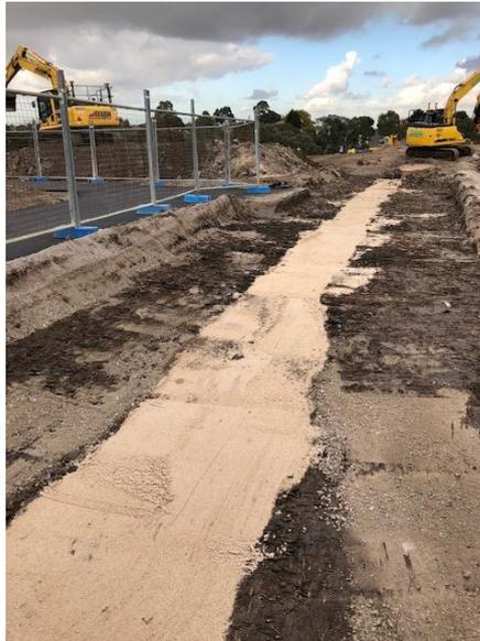
Figure 2 & 3: Backfilling the trench with a sand filter (2) and the sand filter trench completed (3)
