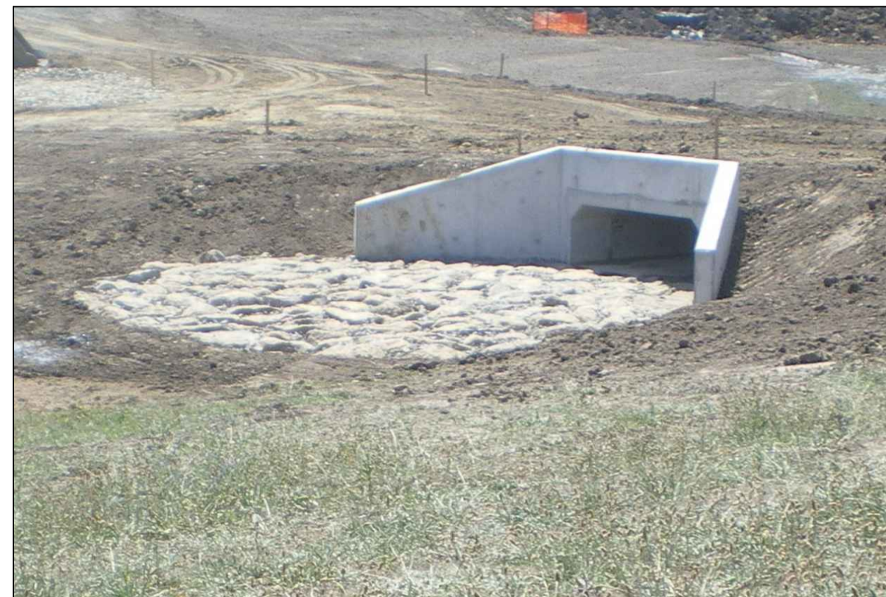
CONCRETE WING WALL PHOTO
