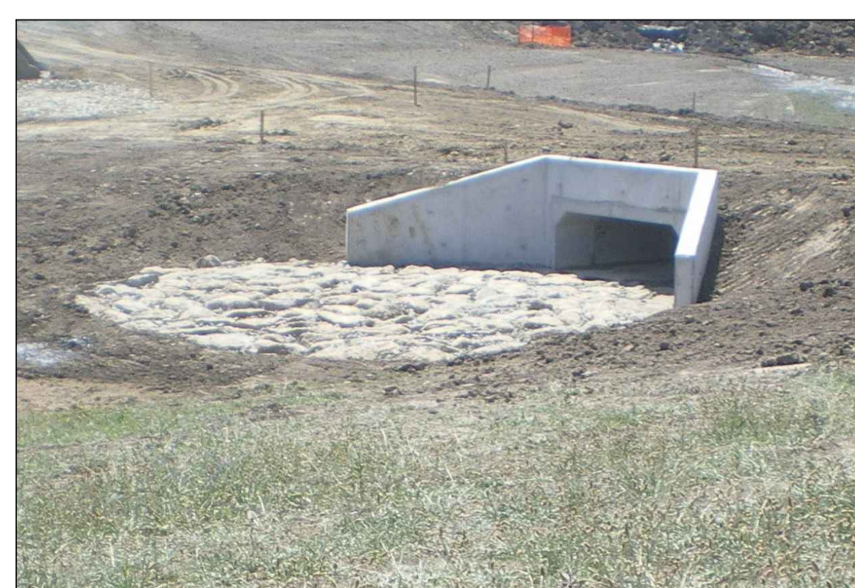
CONCRETE WING WALL PHOTO
