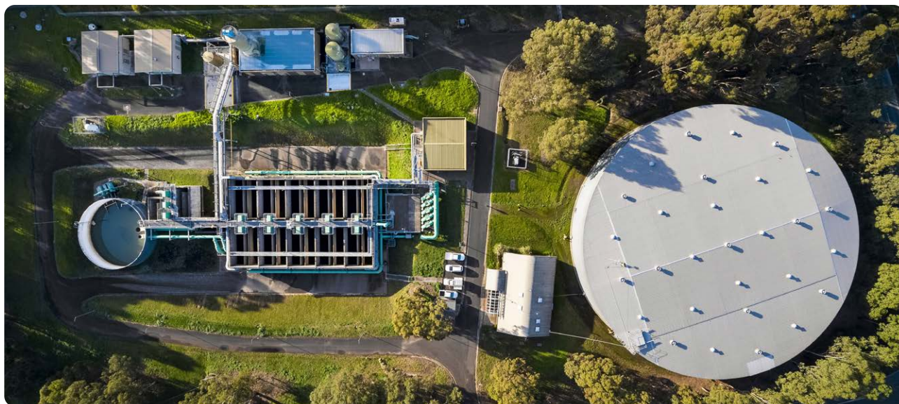
Yan Yean water treatment plant
