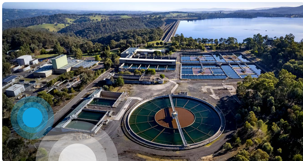
Winneke water treatment plant
