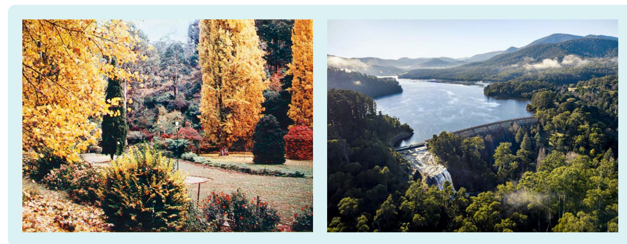
FIGURE 9 • The Maroondah Reservoir park below the dam wall has been enjoyed by the community for nearly 100 years
