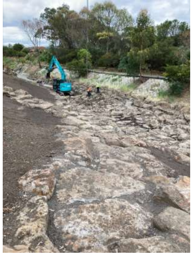
Naturalisation works in progress
