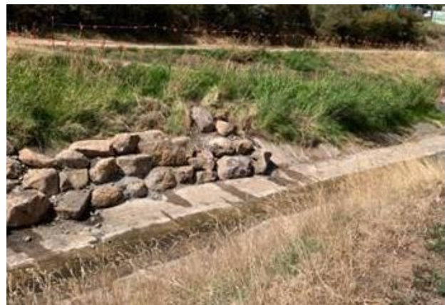
Rockwork lining in progress
