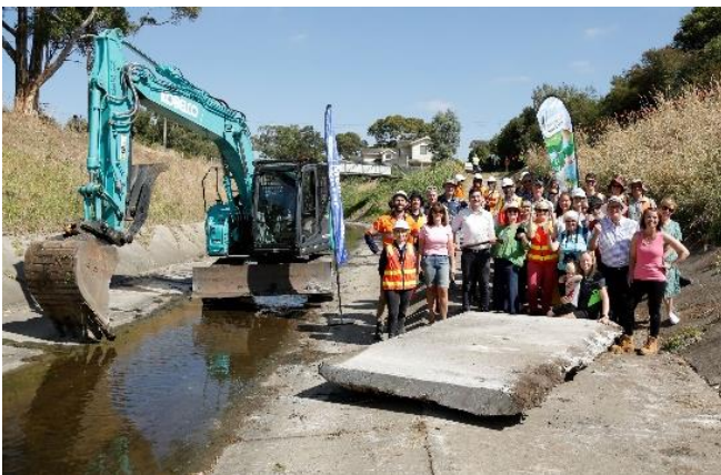
Celebration of first concrete panel removed
