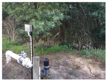
Figure 2: Full flowing pipe meter with Ajenti transmitter
