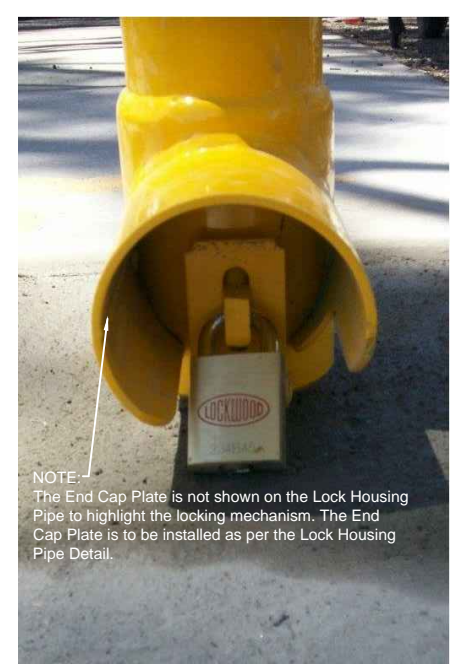
Photo 2 TYPICAL SINGLE LOCK BOLLARD – FRONT VIEW. LOCK MECHANISM (HINGED HASP LIFTED OVER LOCK PLATE STAPLE, THEN PADLOCKED). NOTE: HALF END CAP MISSING, DEMONSTRATION ONLY
