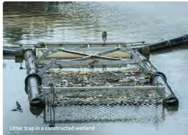
Litter trap in a constructed wetland
