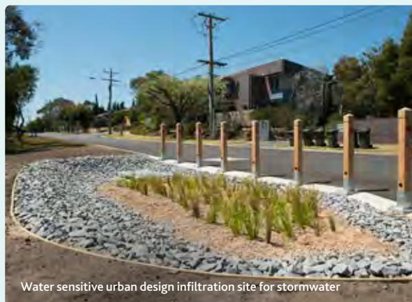
Water sensitive urban design infiltration site for stormwater
