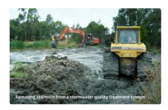
Constructed wetlands are a series of shallow, densely planted ponds that help filter water through physical and biological processes. They replicate nature's way of treating and removing pollutants from stormwater before it enters creeks, rivers and bays.
