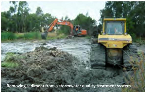
Removing sediment from a stormwater quality treatment system
