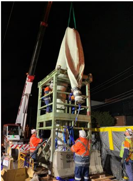
Inserting the 185m liner into manhole 1
