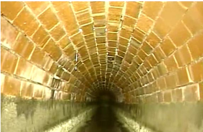
Existing brick sewer
