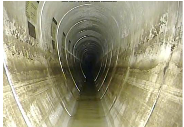
Newly relined sewer
