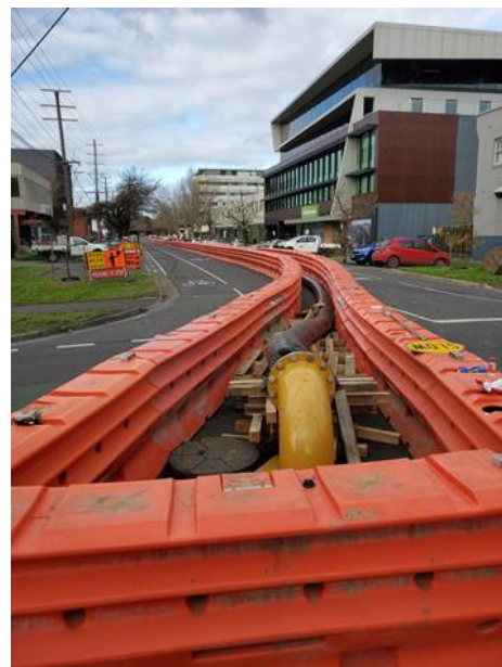
Richmond bypass on Palmer Street
