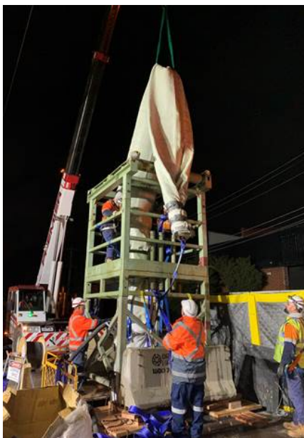
Installation of the 185m long CIPP liner
