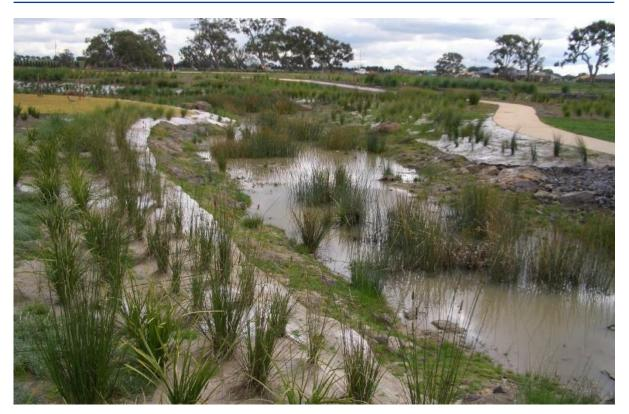
Figure 44 - Example of a recently planted constructed waterway, showing in stream, bank and riparian plantings
