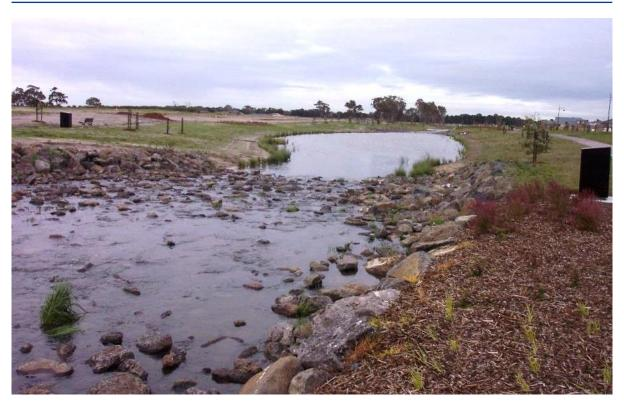
Figure 14 - Example of a constructed pool-riffle sequence
