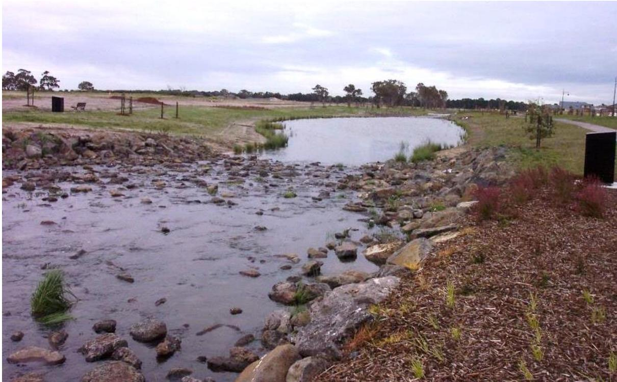
Figure 14 - Example of a constructed pool-riffle sequence
