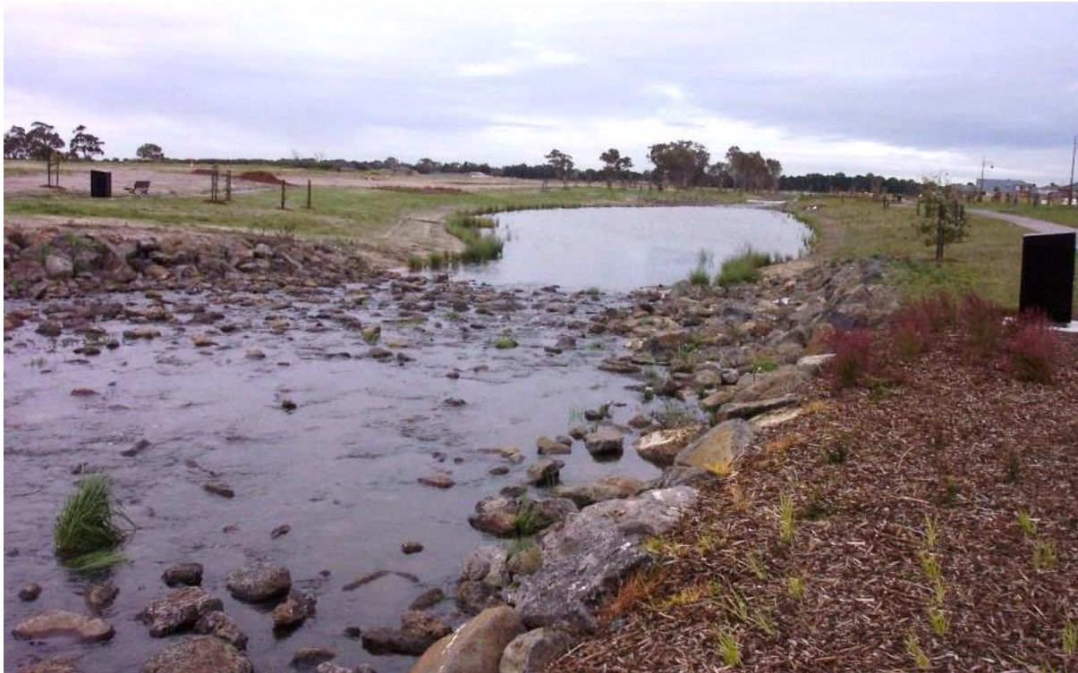
Figure 14 - Example of a constructed pool-riffle sequence
