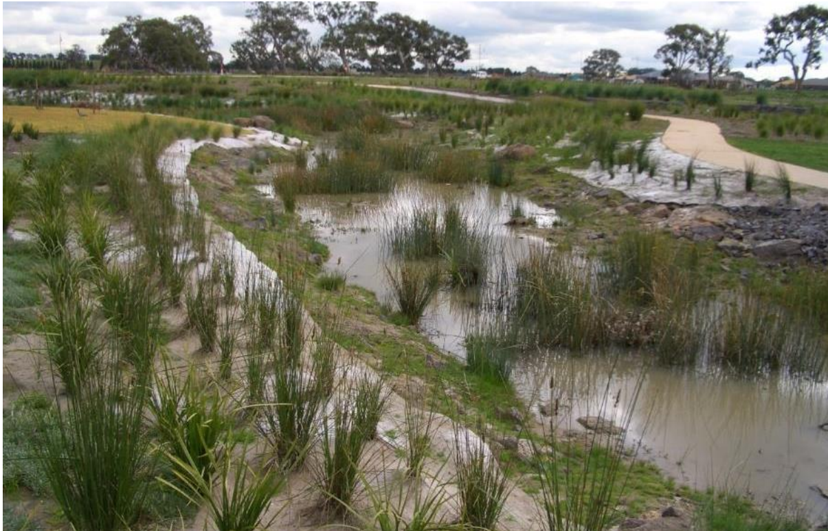
Figure 44 - Example of a recently planted constructed waterway, showing in stream, bank and riparian plantings
