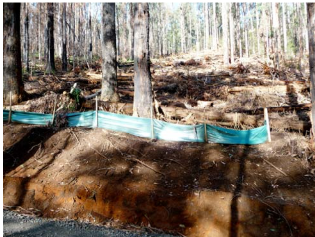
Rehabilitated fire-break with a silt fence
