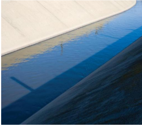
Western Treatment Plant channels
