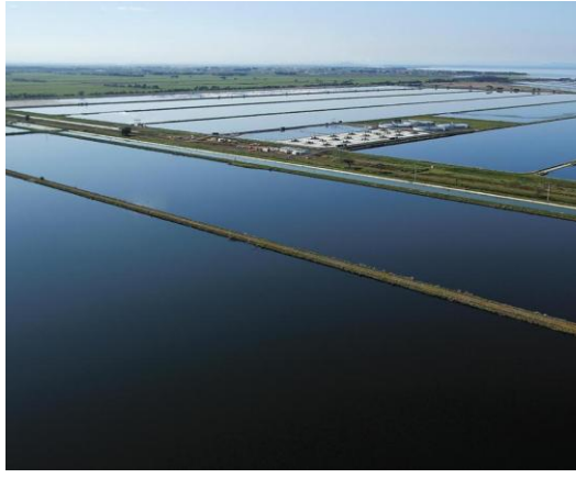
Western Treatment Plant lagoons
