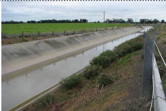
Effluent entering Western Treatment Plant
