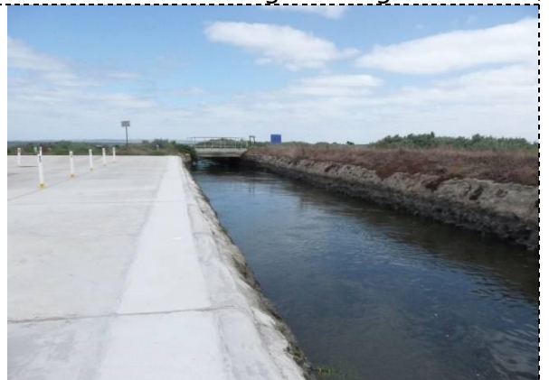
Open channel leading out to Port Phillip Bay
