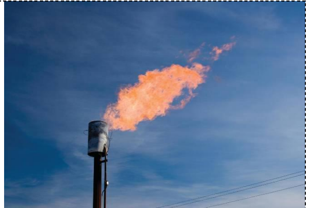
Excess methane gas being burned
