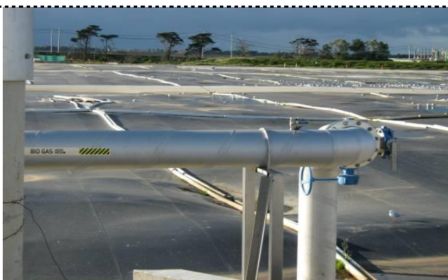
Ponds covered with black plastic to capture methane
