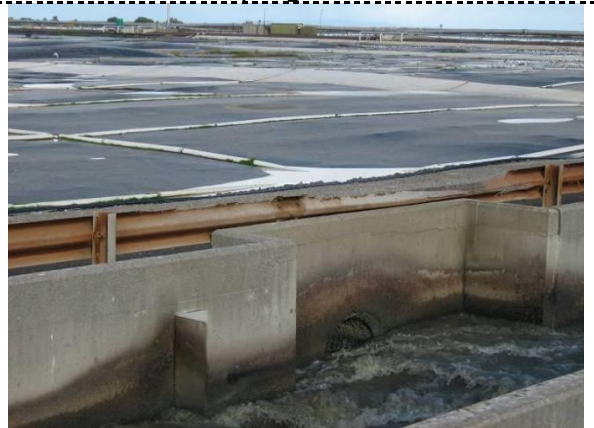
Ponds where sedimentation takes place
