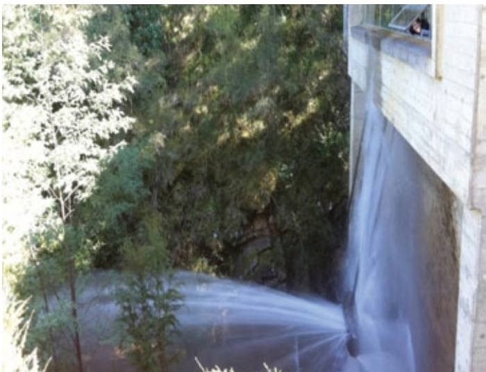
Water being released from the Upper Yarra Reservoir on 19 September 2011
