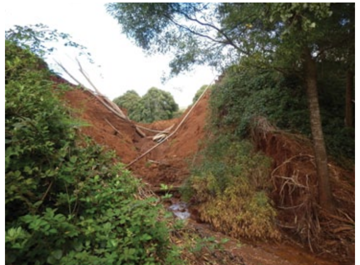
Failed dam in Gembrook Area
