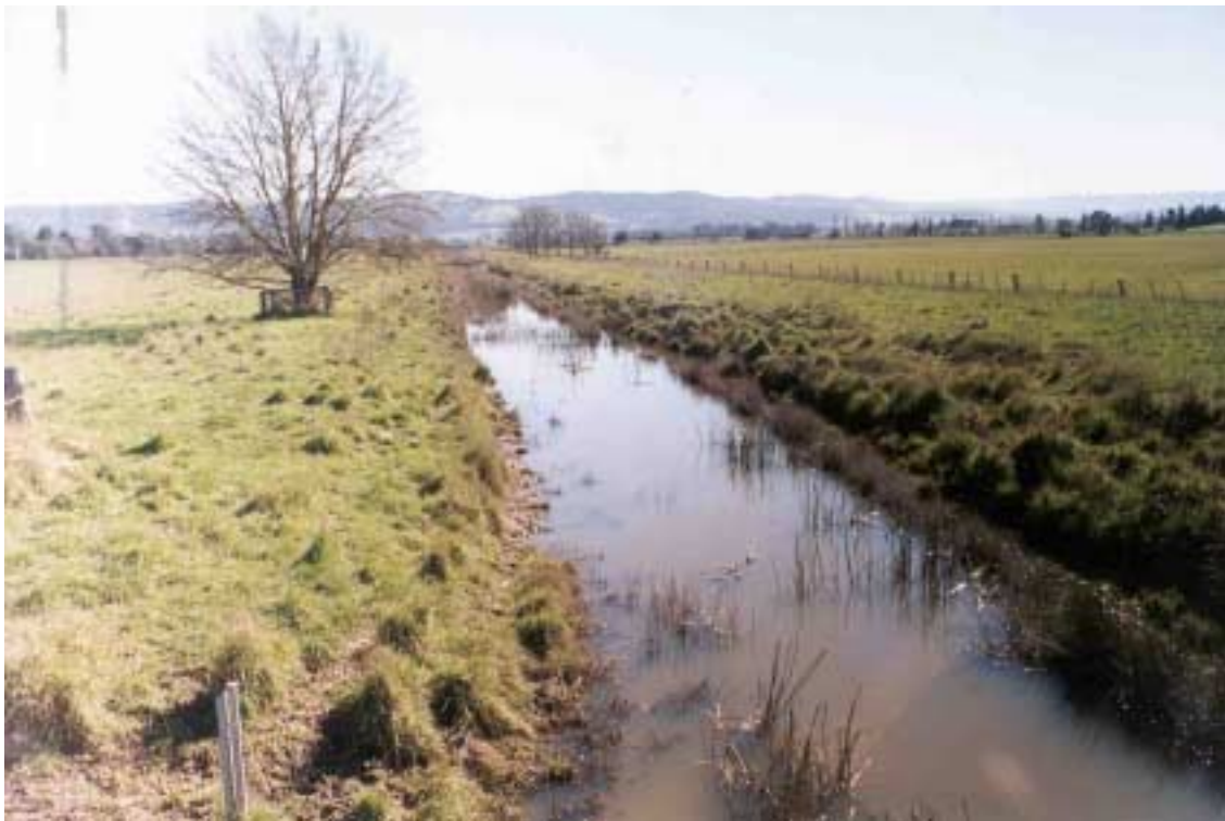
Figure 6-4. Stringybark Creek downstream of bridge on Melba Highway.
