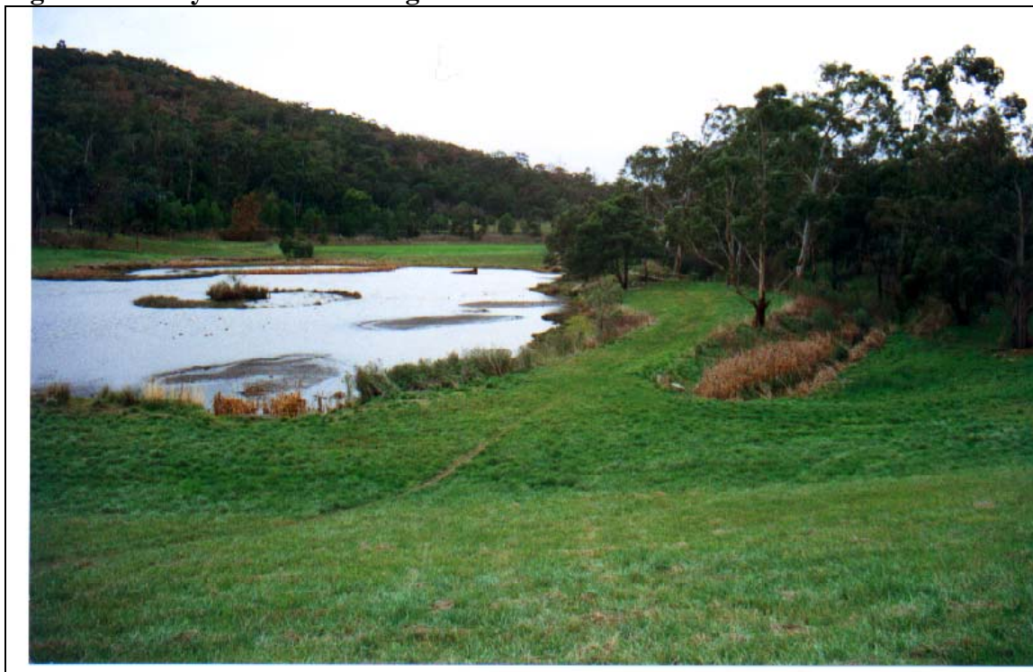
Figure 9: Ferny Creek Retarding Basin
