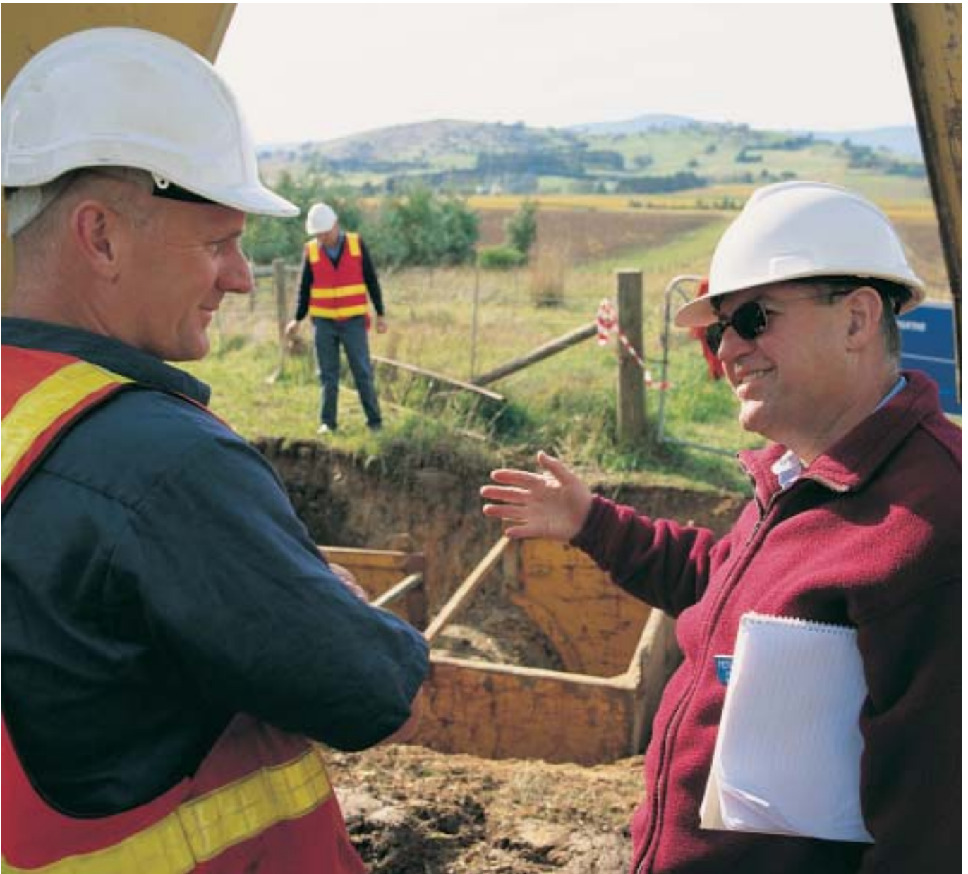
A site safety audit at Yarra Glen for the pipe repair team.
