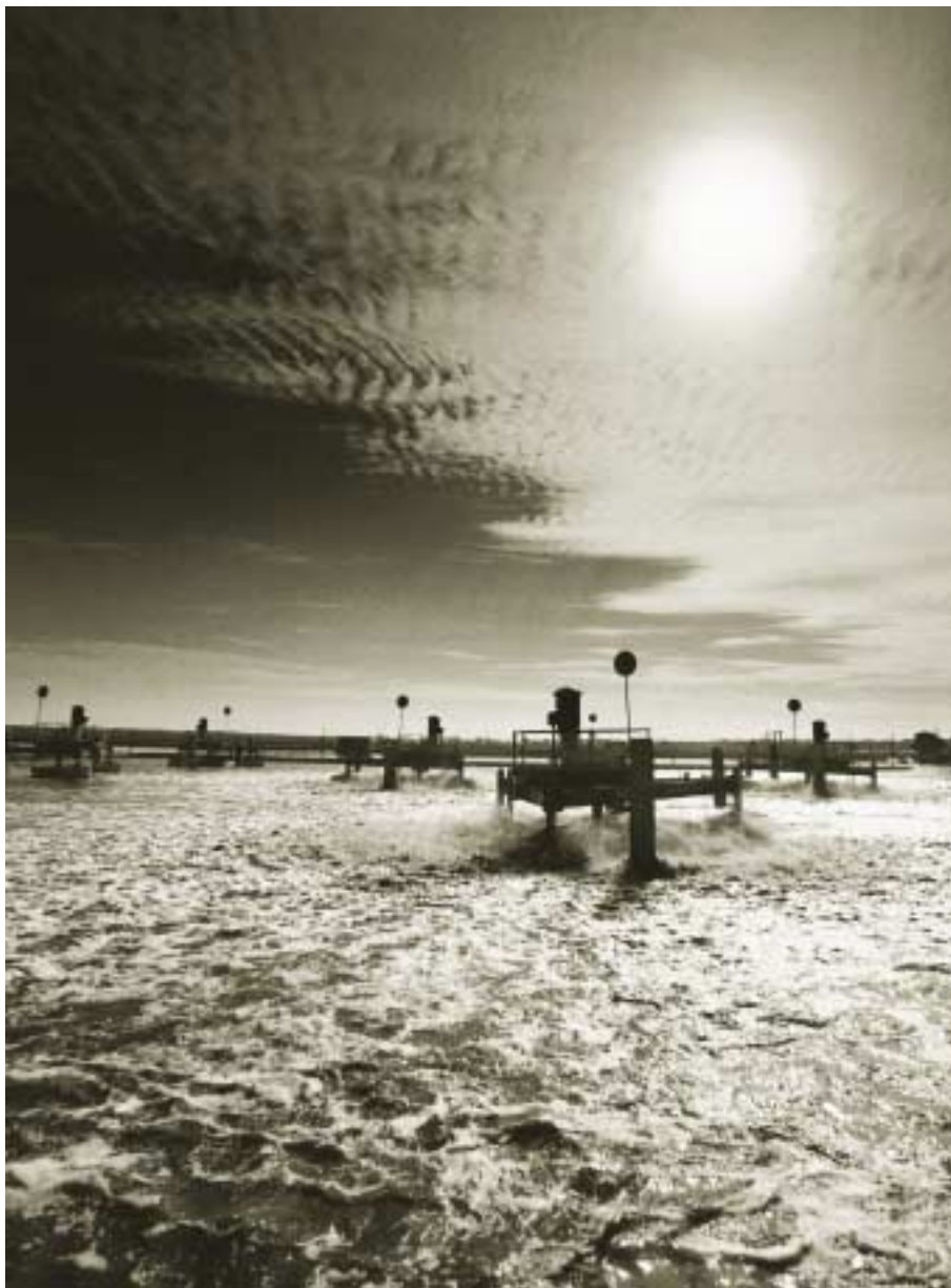
Aerators at work in the lagoon system at our Western Treatment Plant.
