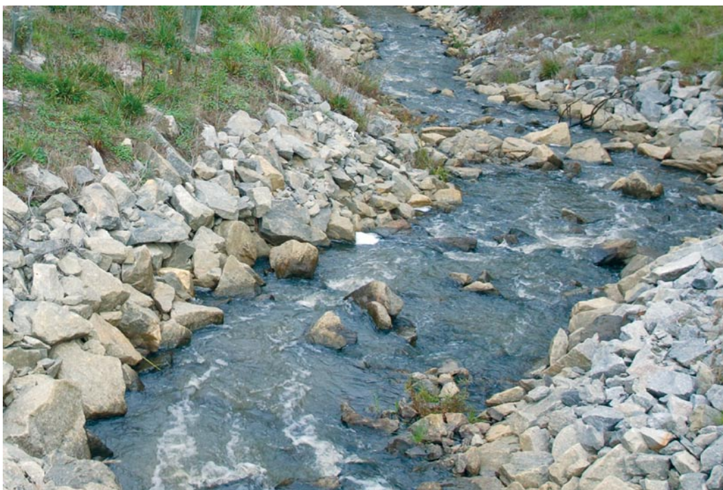
Cardinia Creek fishway at Clyde North.
