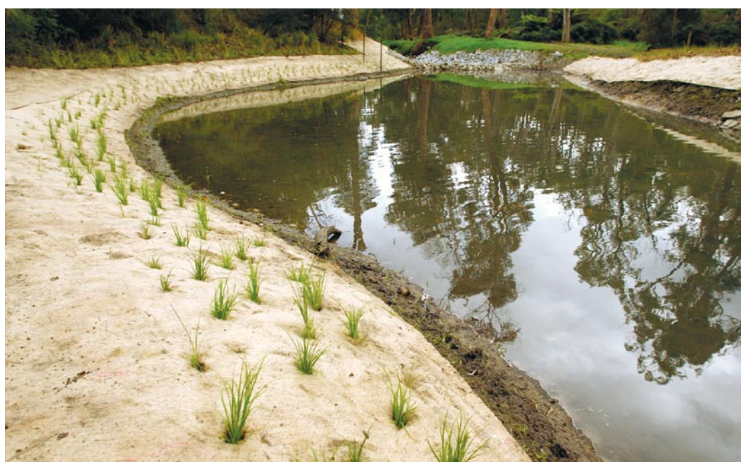
Rehabilitation works along Old Joe's Creek in Boronia.
