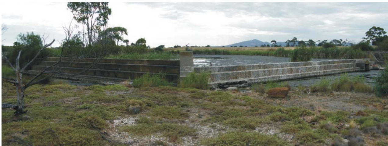
Weir on Little River near Little River township.
