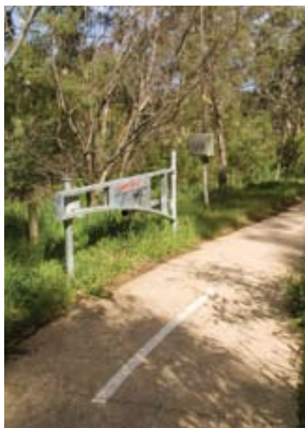
FLOOD ACTIVATED BOOM GATE
