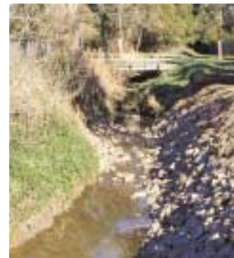
Streamlined: Brushy Creek after restoration
