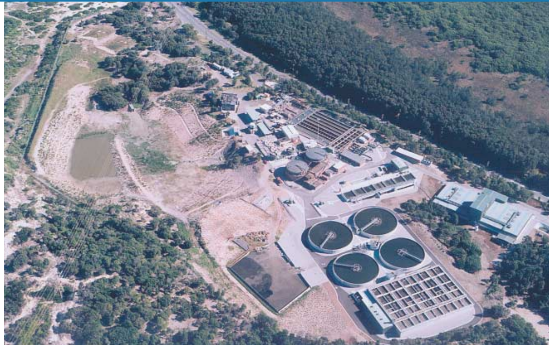
ABOVE Setting a new benchmark: The Cronulla sewage treatment plant, which is believed to be the largest plant of its kind to discharge such high quality effluent to the ocean
