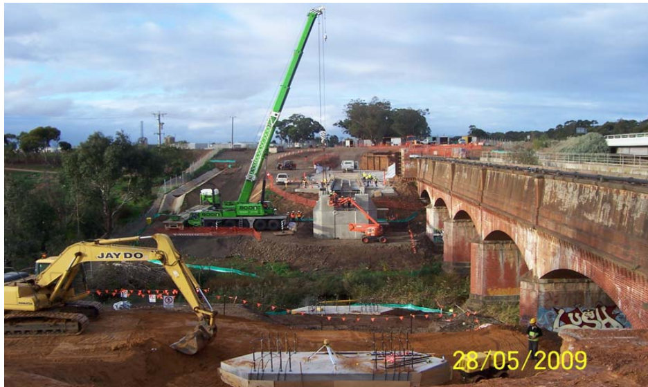
1. Site works looking towards Melbourne.
