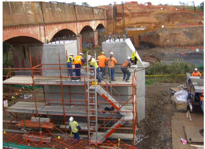
3. Final top unit installation
