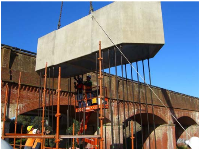
2. First base unit installation
