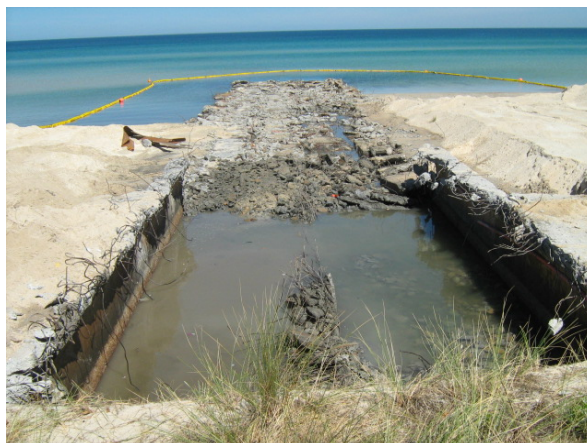
It didn't take long to demolish the old structure
