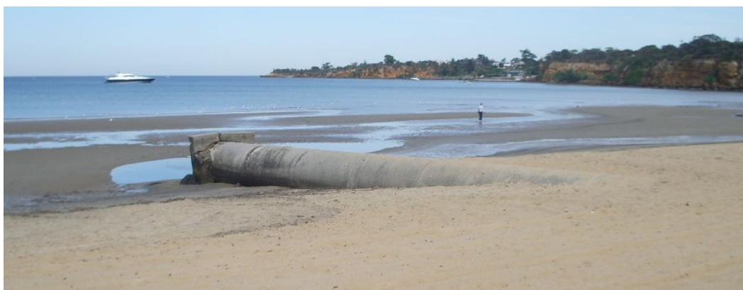
Melbourne Water's Marina Road drain which is to be upgraded
