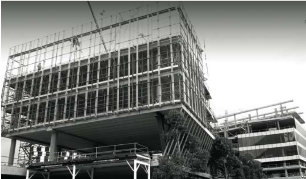
Left: Construction of Melbourne Water's new head office
