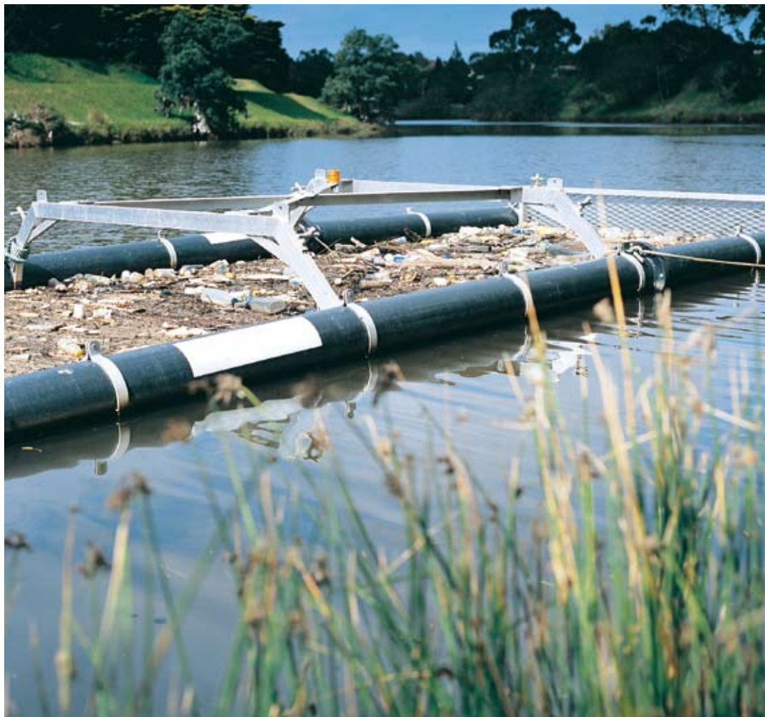
A litter trap in the Yarra River at Burnley captures rubbish washed from our streets into the stormwater system when it rains.
