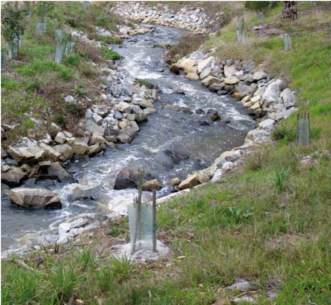
Cardinia Creek Fishway at Clyde North
