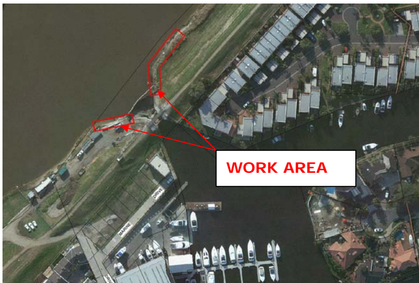
Town Centre Tidal Gate. Melways reference 97H5
